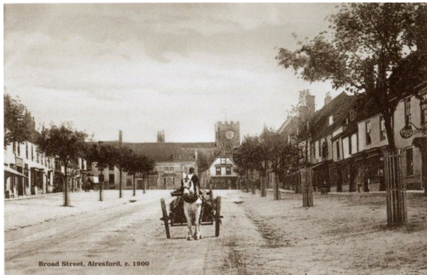
Figure 4. Broad Street sidings, trees and guards in 1900 (looking south with St John's Church clock tower in the centre background and New Alresford Town Hall to its left).
